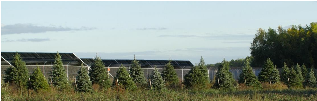
Vegetative screening will grow to obscure panels from the road and nearby homes, when desired. Photo Credit: Borrego Solar
