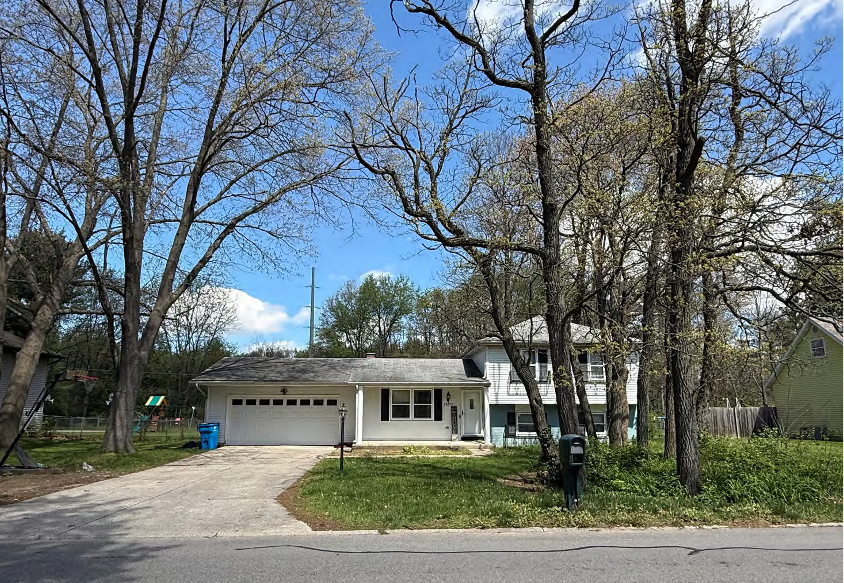
Subject property facing north
