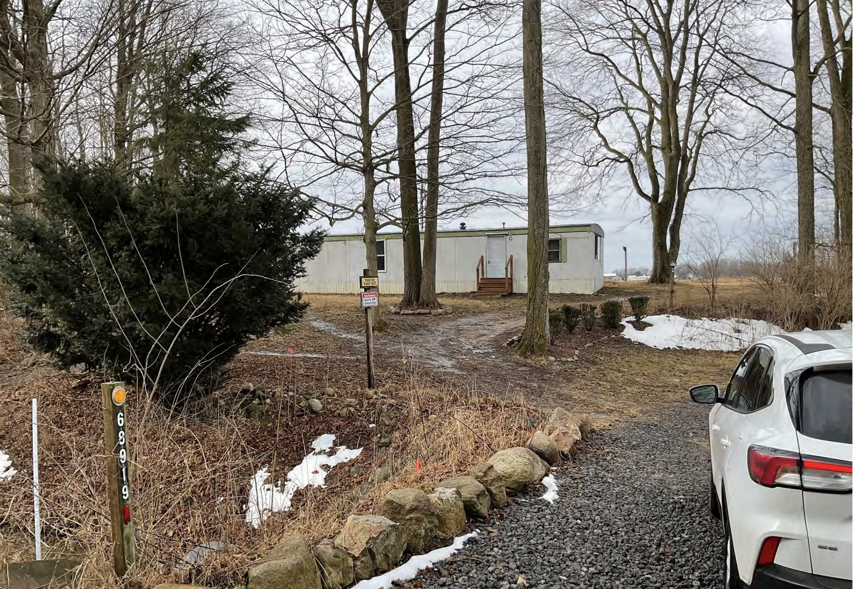
Subject property, facing west
