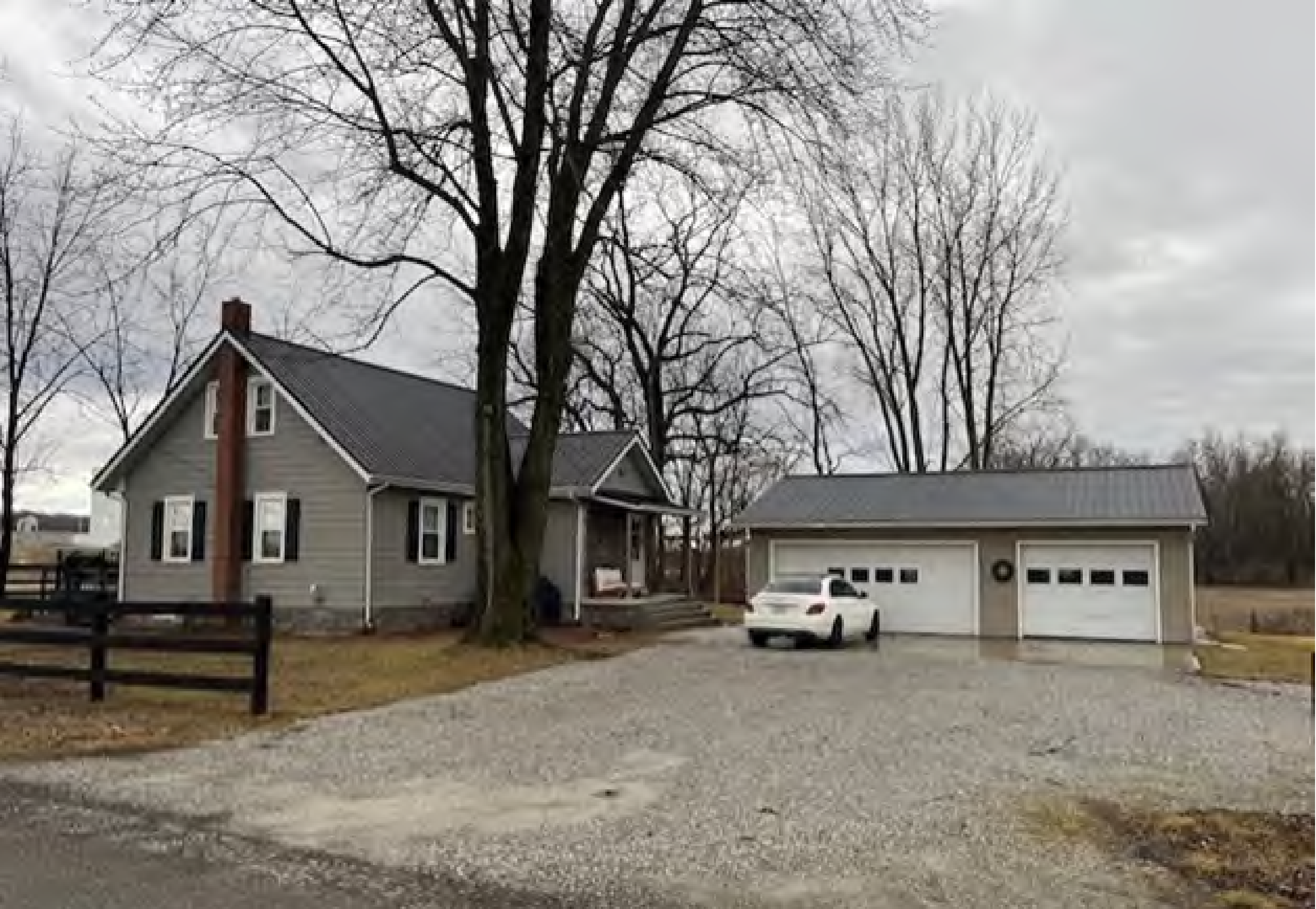
Subject property facing south
