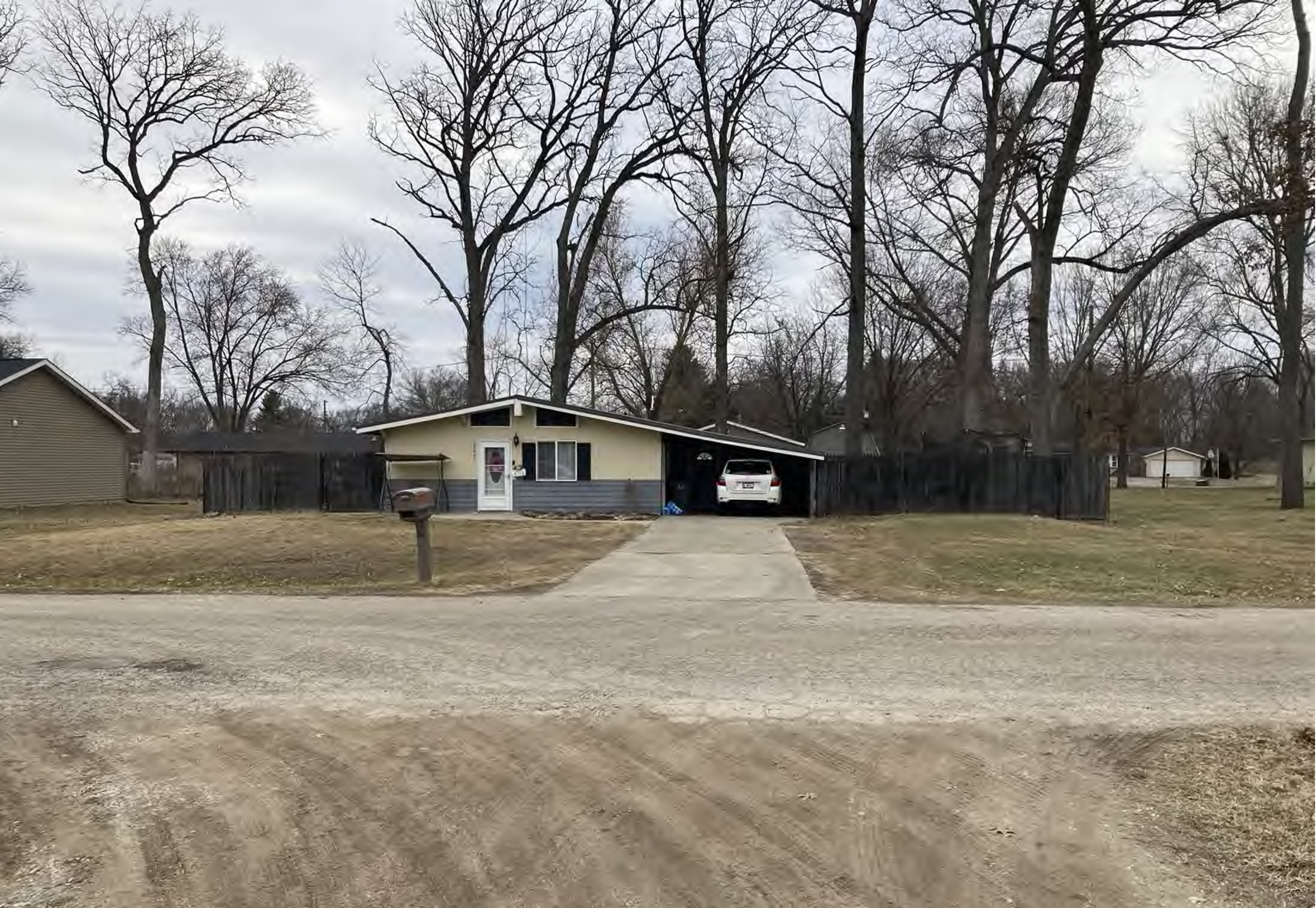
Facing north at entrance
