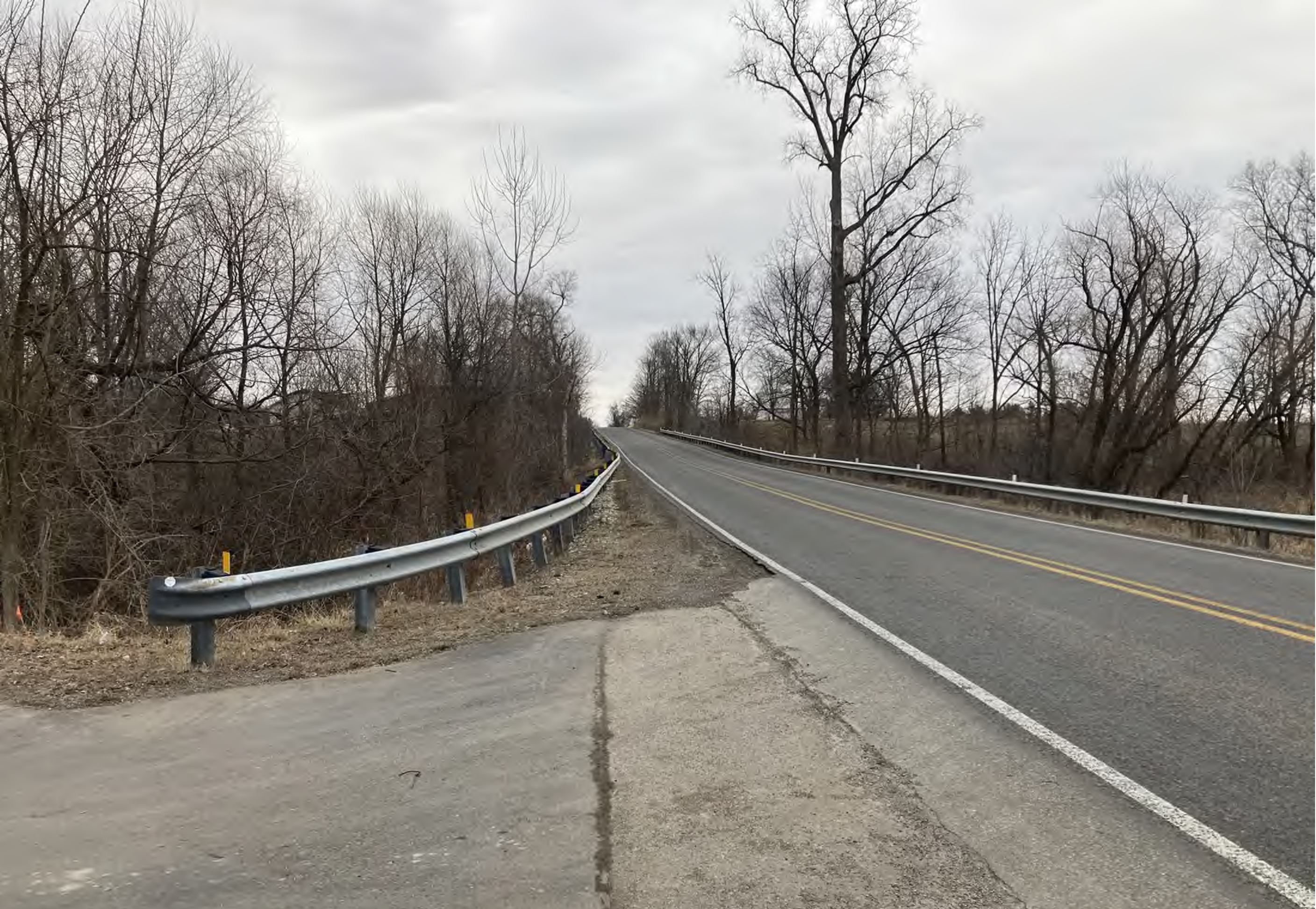
Facing east at entrance
