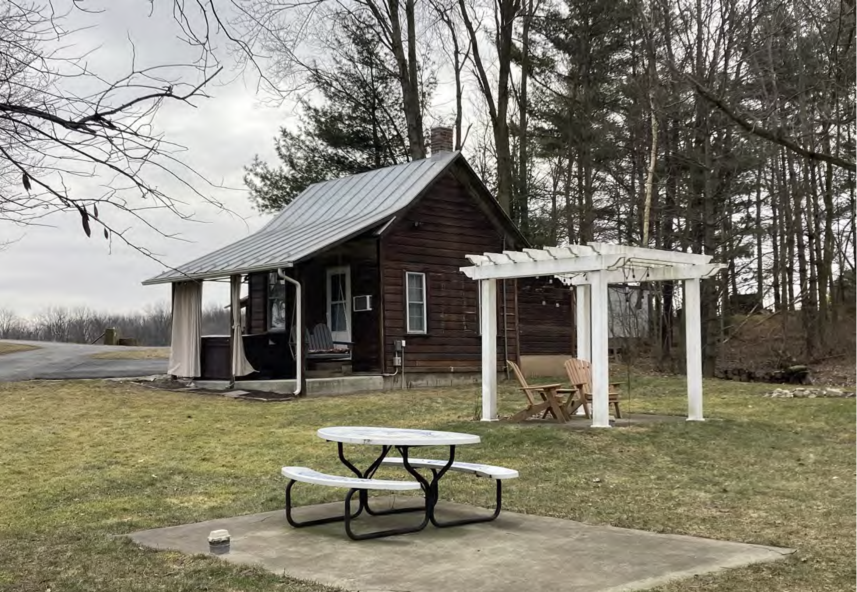
Cottage guest house
