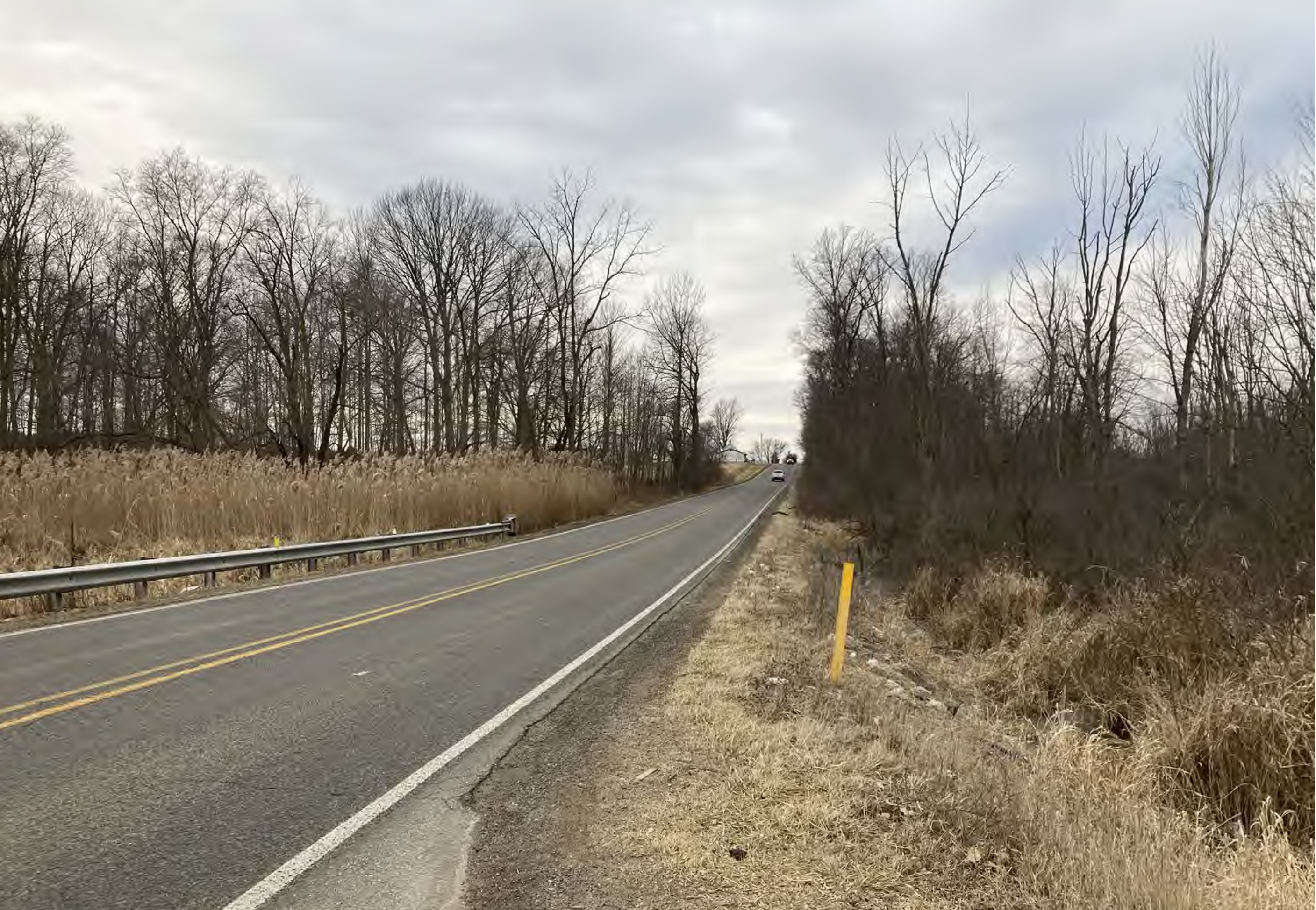
Facing west at entrance
