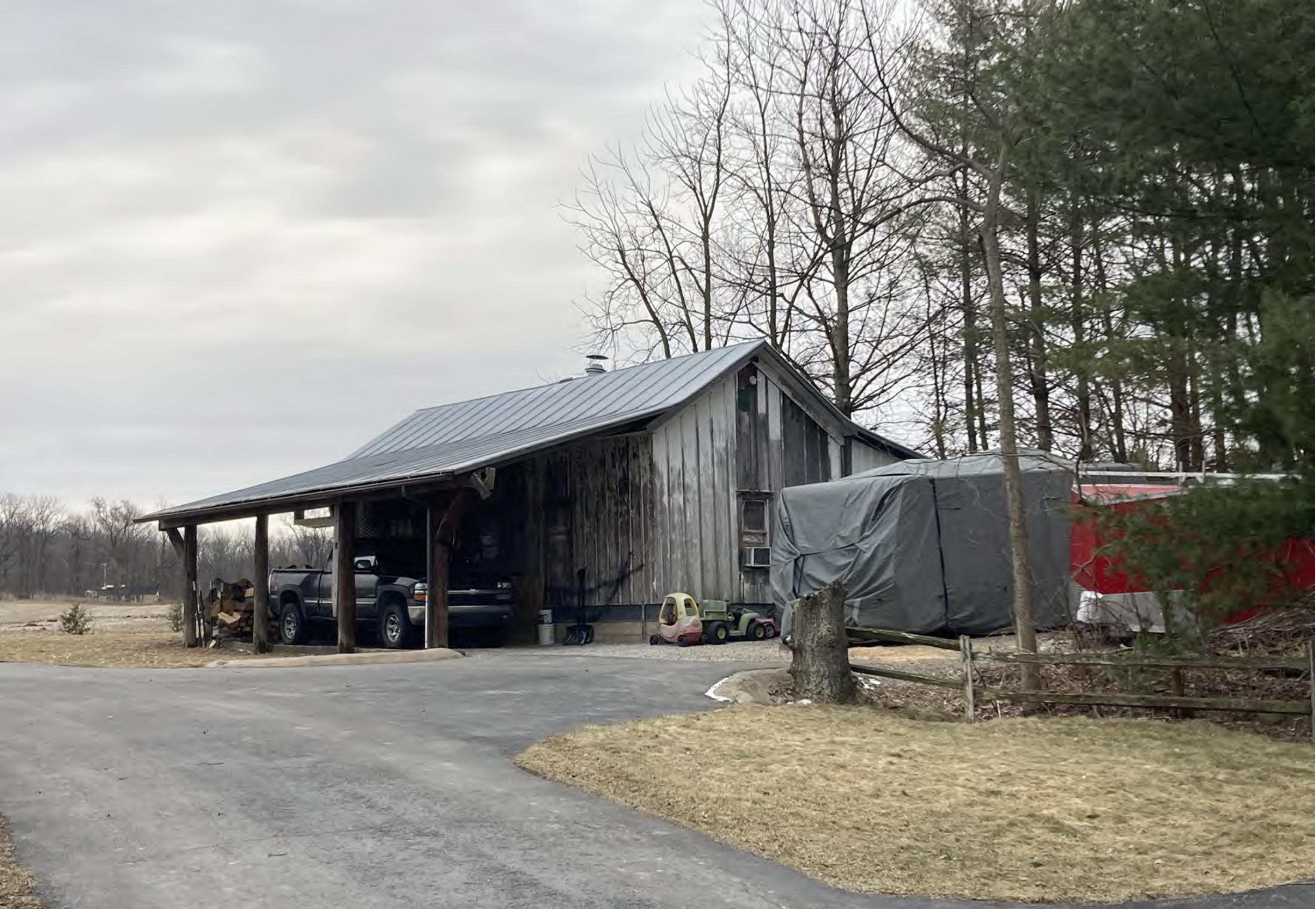
Accessory building (shop)
