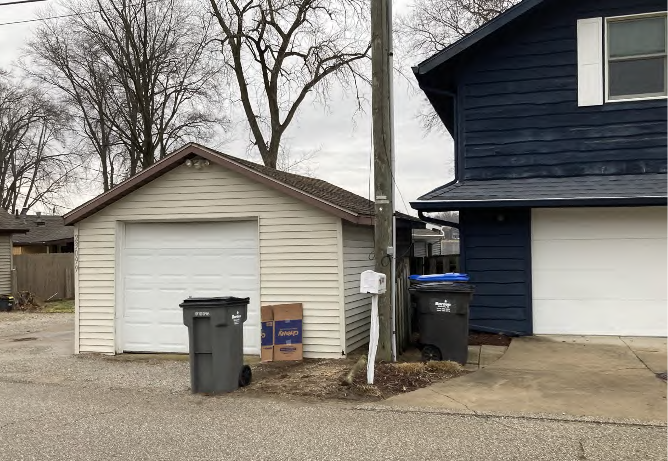
Subject property, Southeast side
