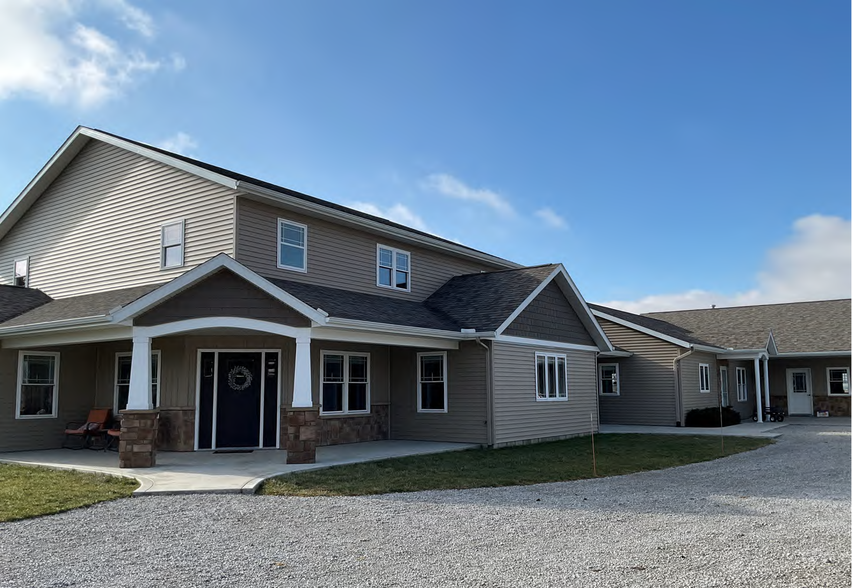
Subject property, facing West
