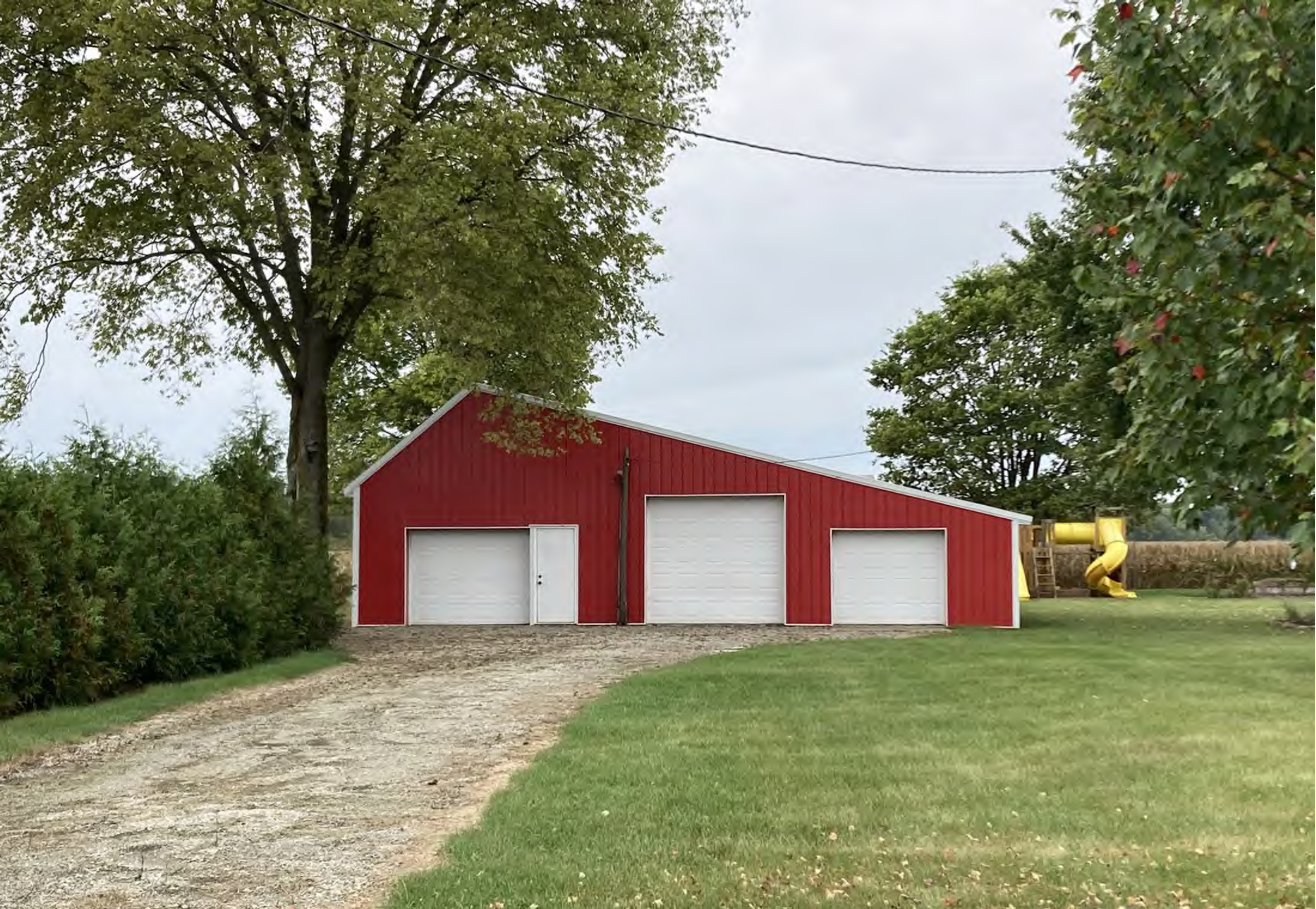
Existing accessory structure
