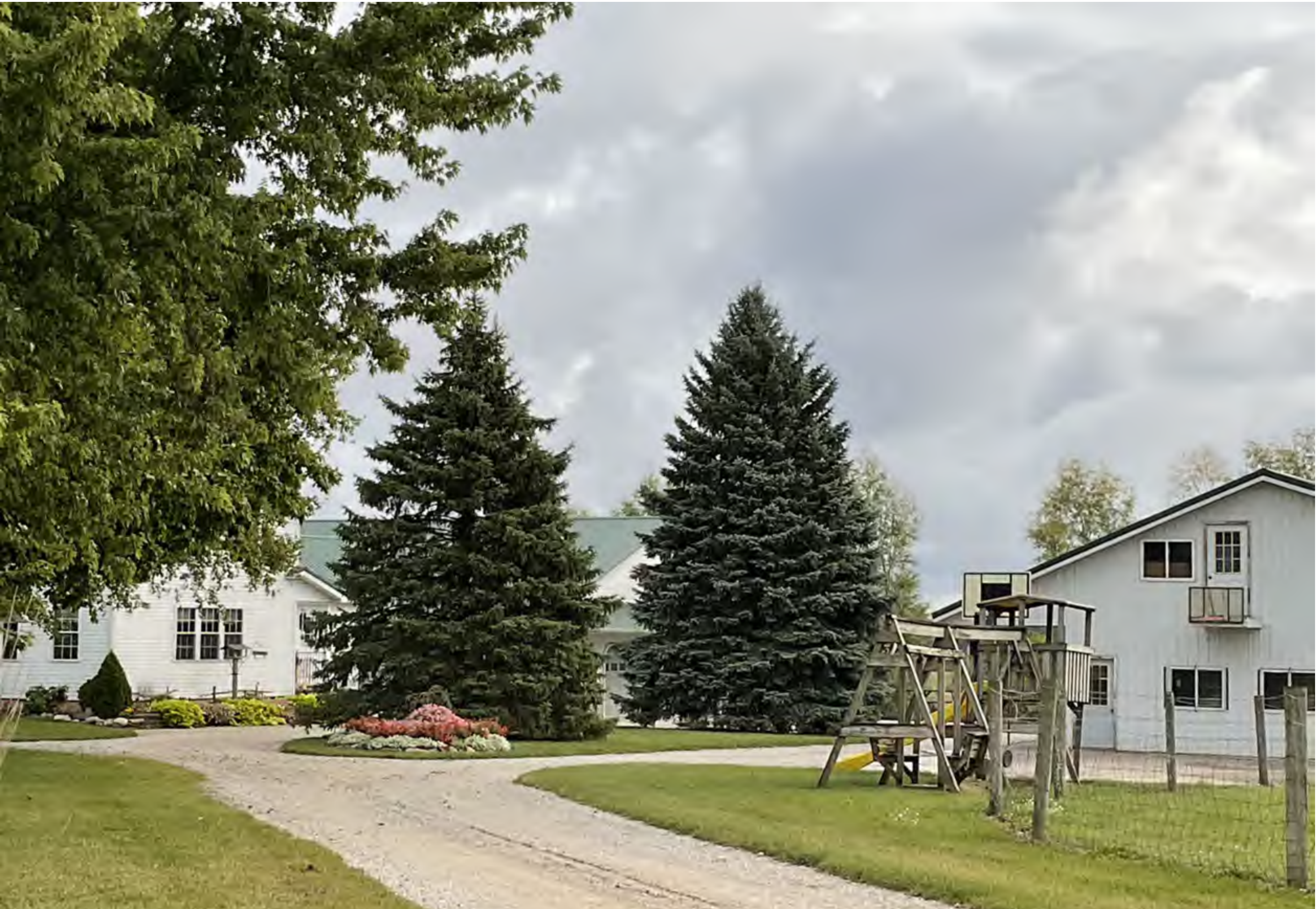
Subject property (residence & garage in foreground)
