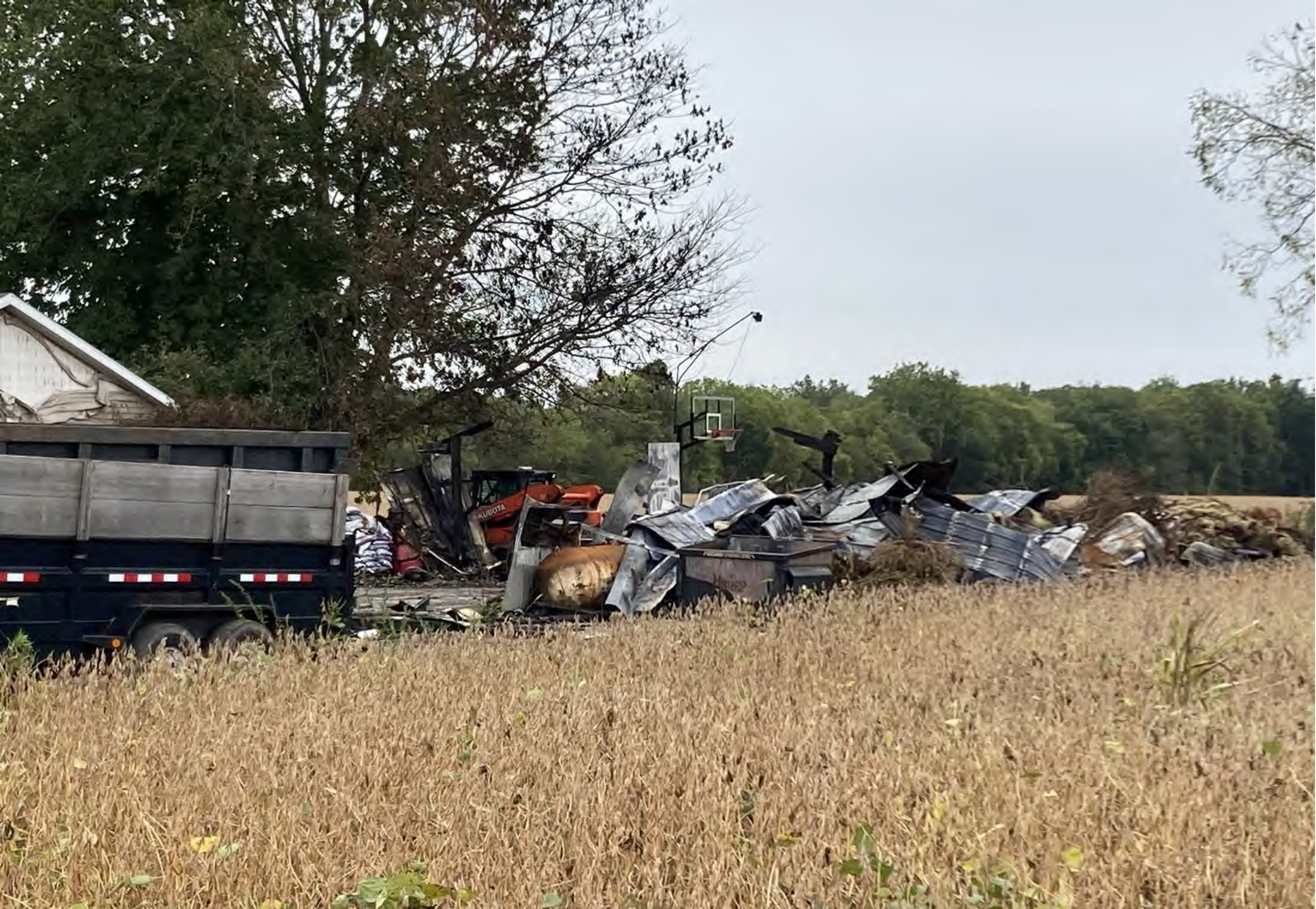
Demolished building in process of removal
