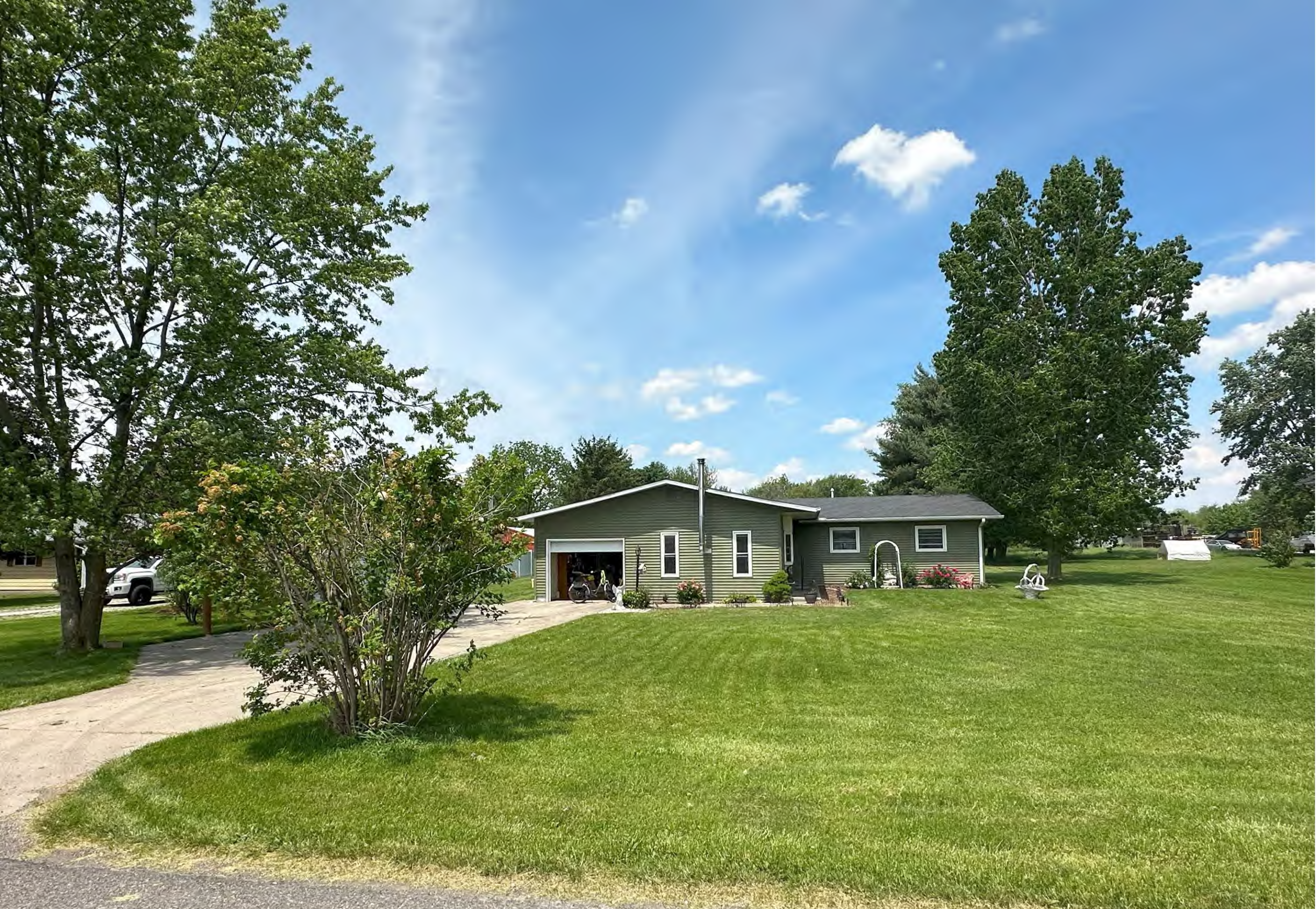
Looking north towards subject property
