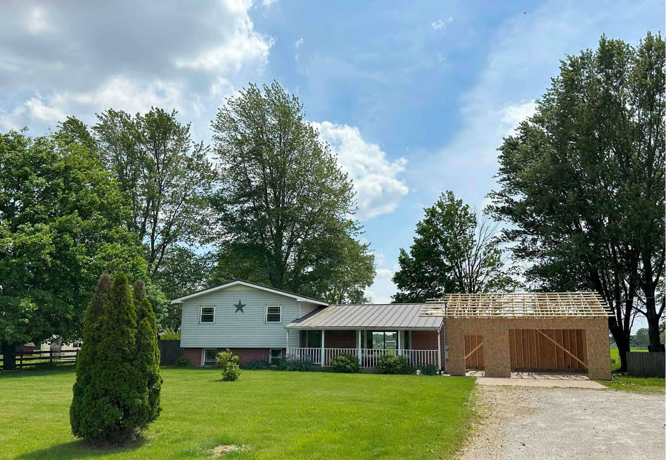
Looking south toward subject property
