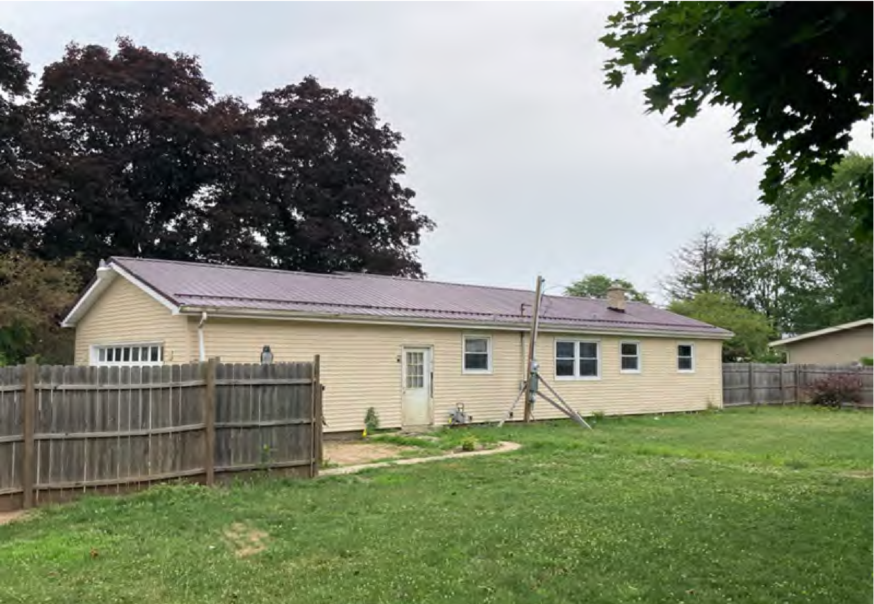
Rear of Subject Property
