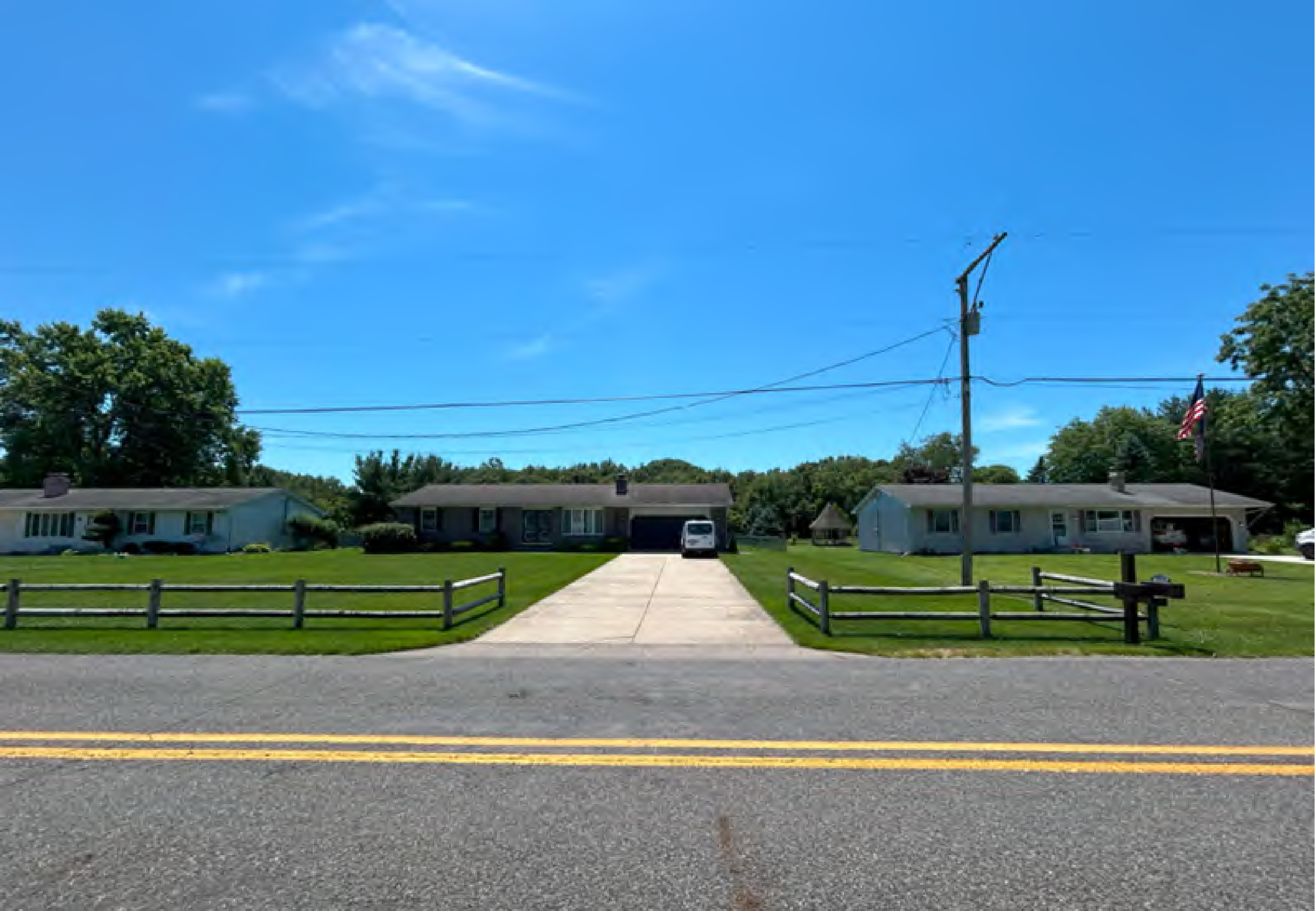
Subject property with current residence (west)
