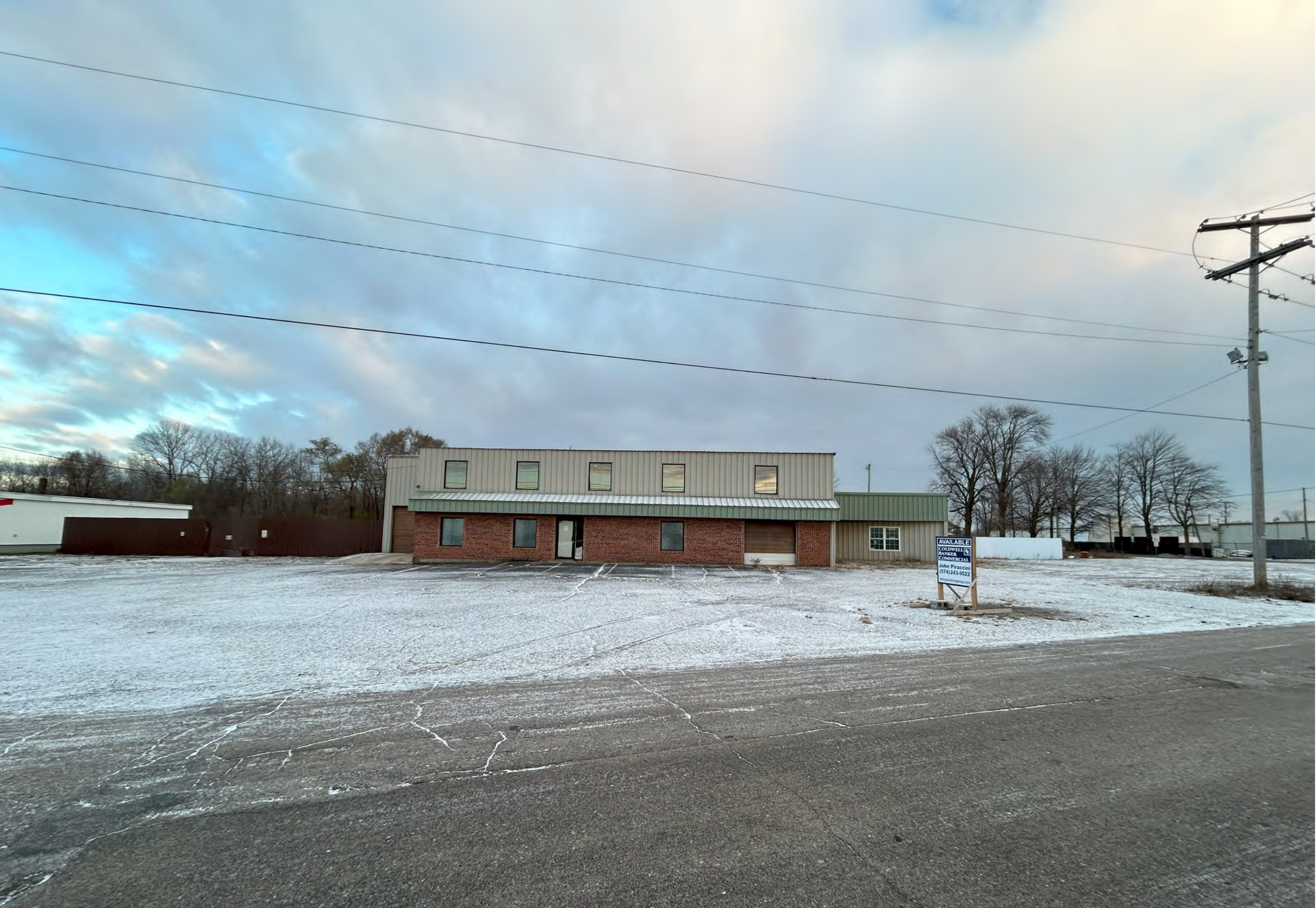
Subject property, facing North
