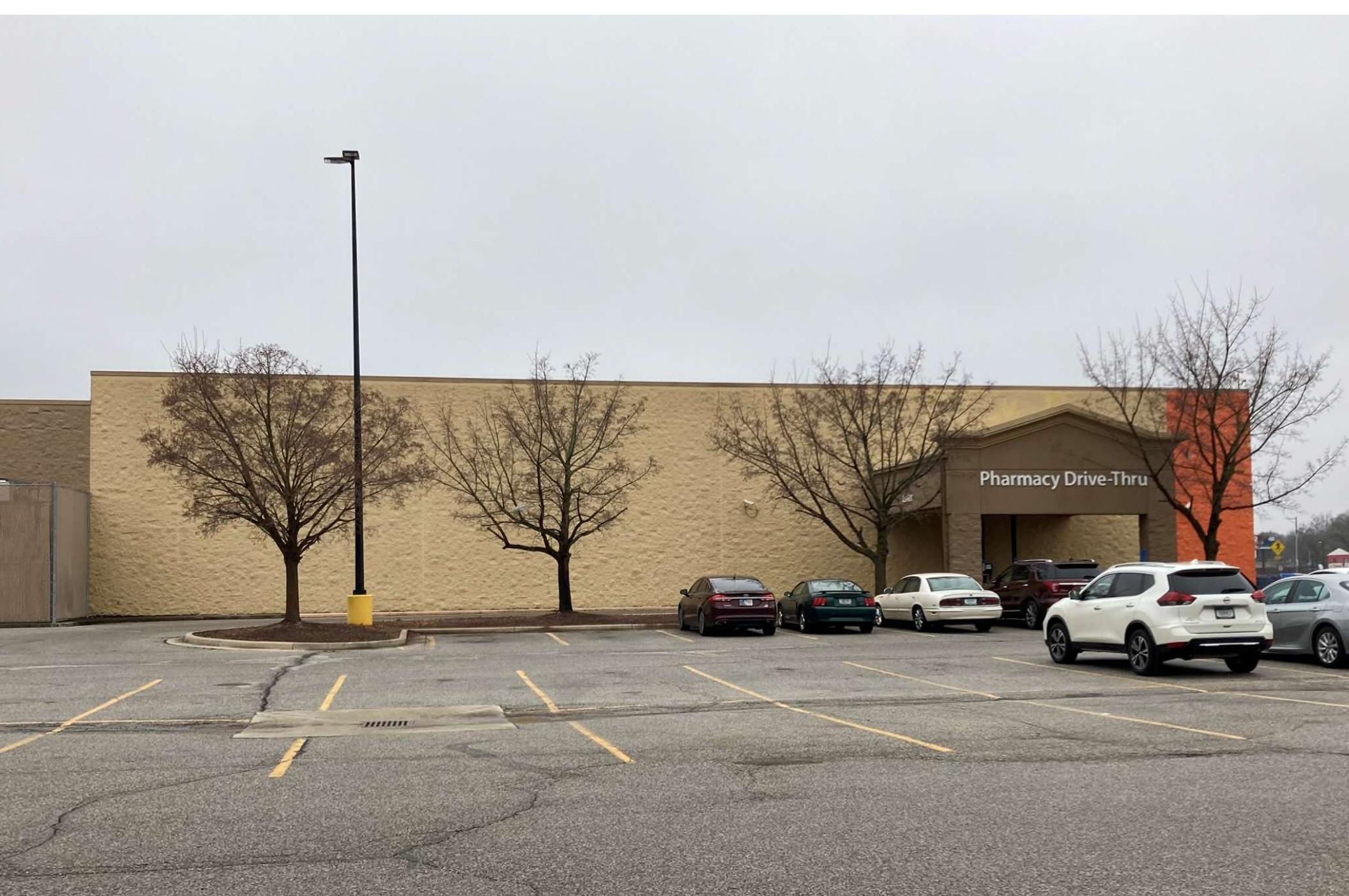
East side of the building
