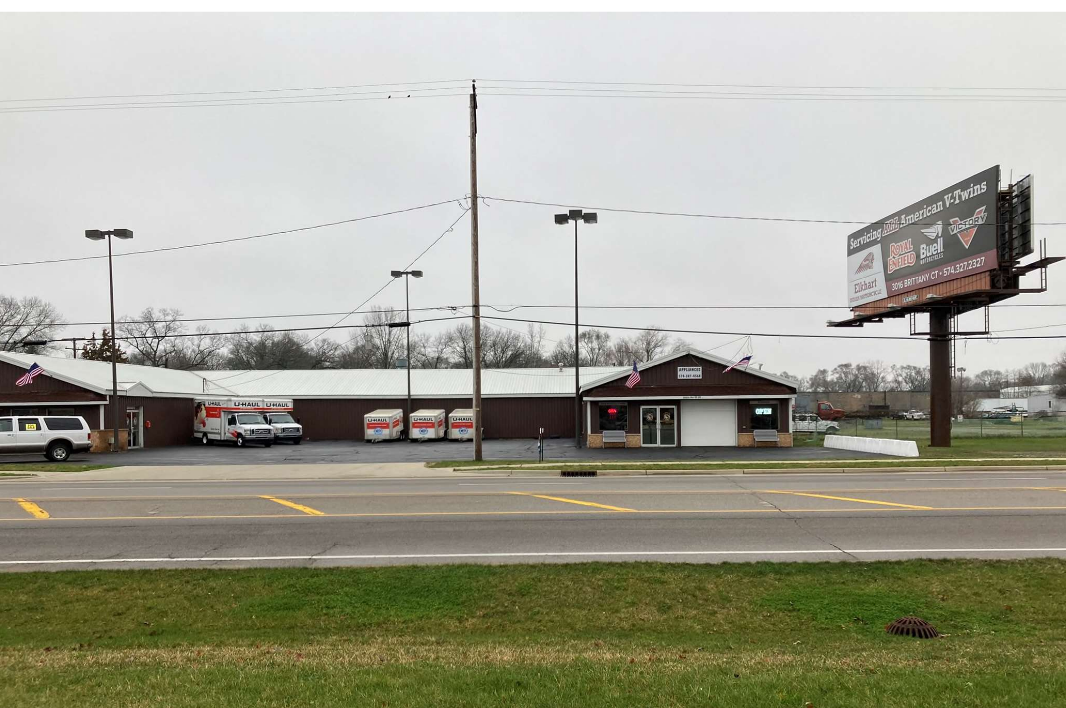
Facing north across Old US 20
