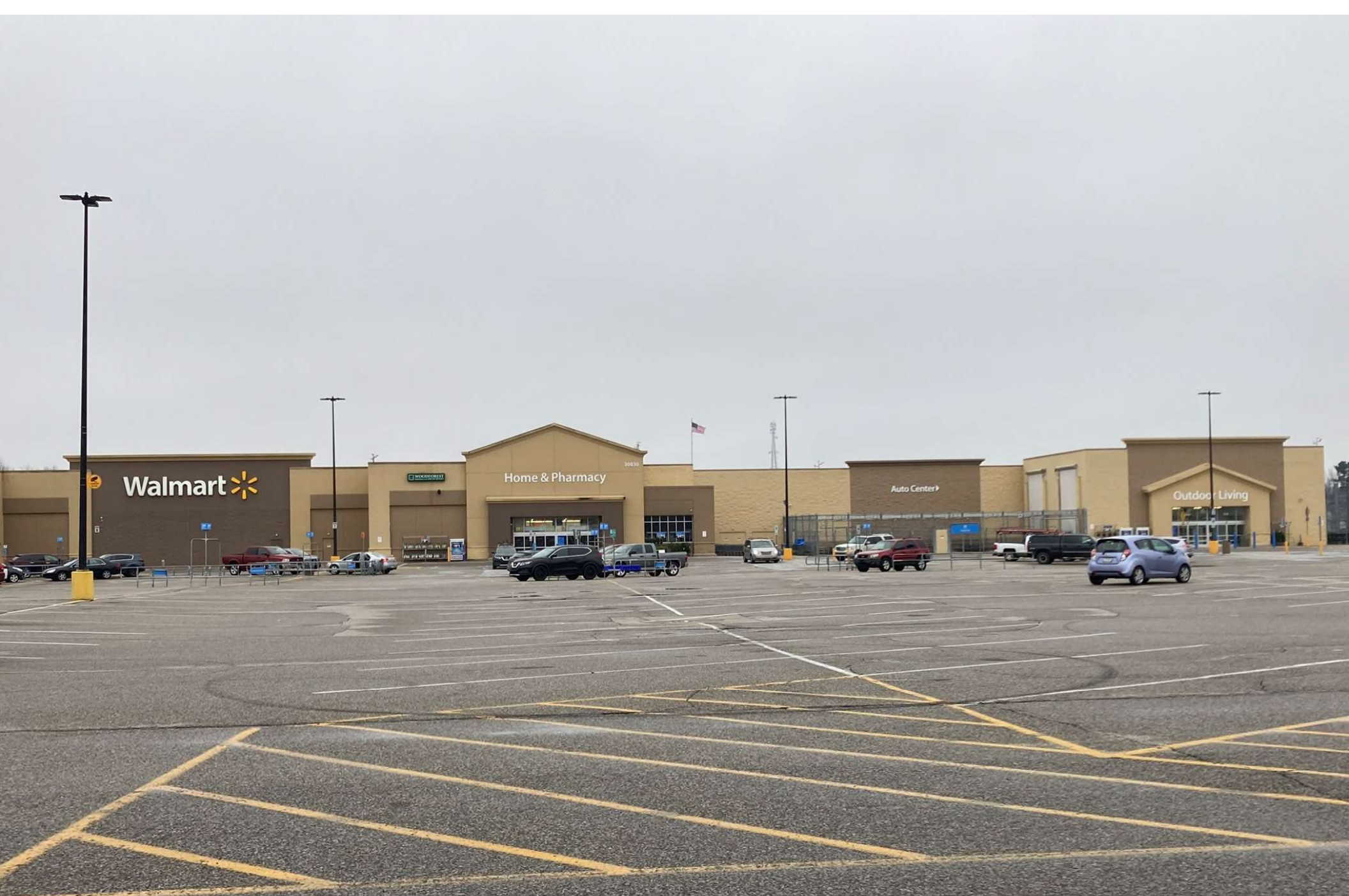
North side of the building, west end
