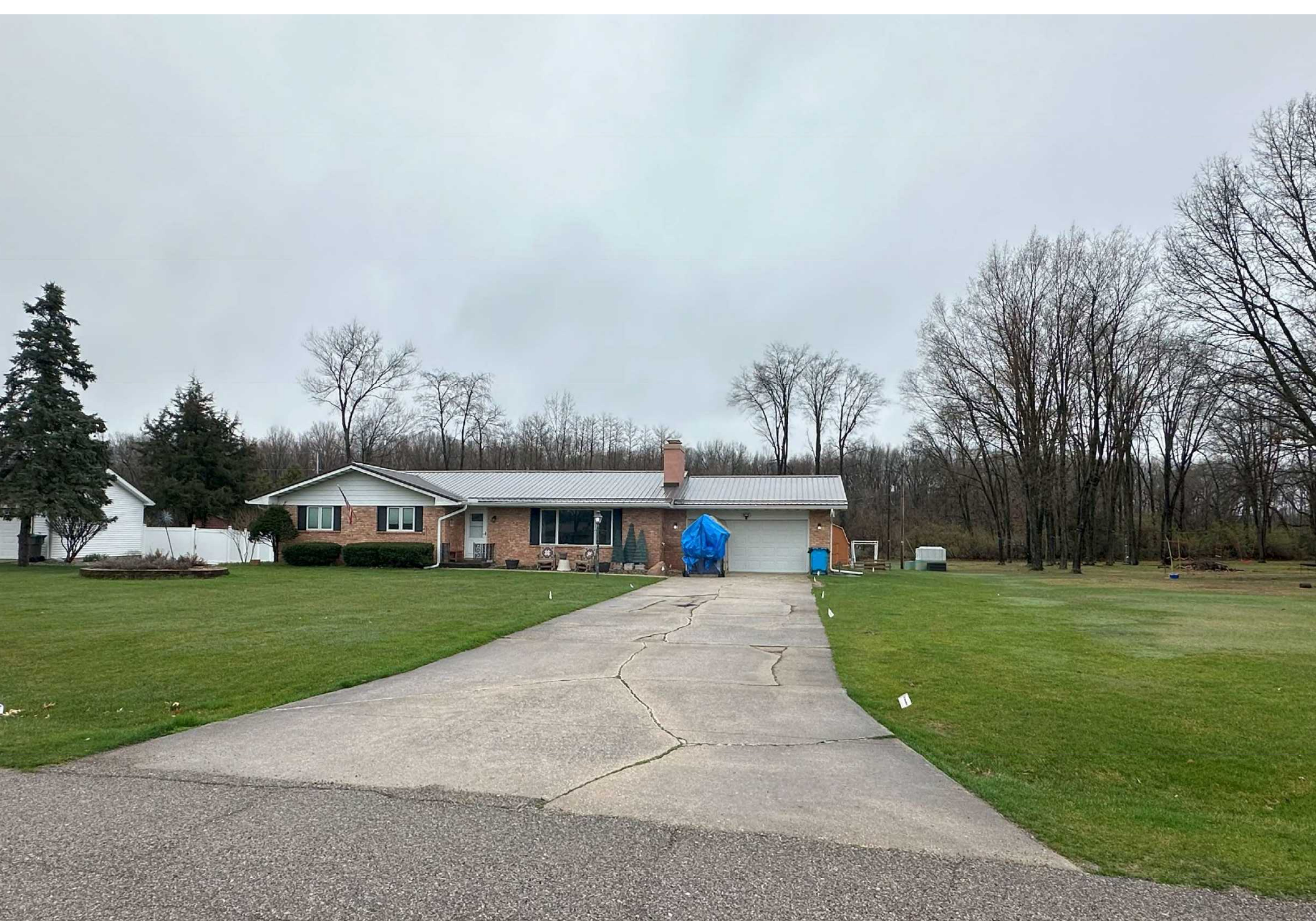
Looking south toward subject property
