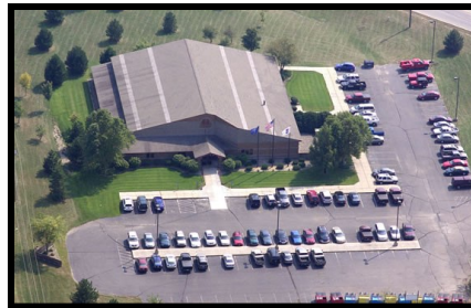
Aerial photograph of the Elkhart County, IN Department of Public Services building
